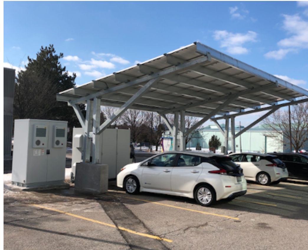
Figure 21. Deployment of residential bidirectional charger.
